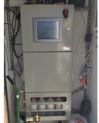
California American Water installed AMS's online, MetalGuard Cr(VI) analyzers, which allowed it to monitor and address critical steps in its remediation process.
