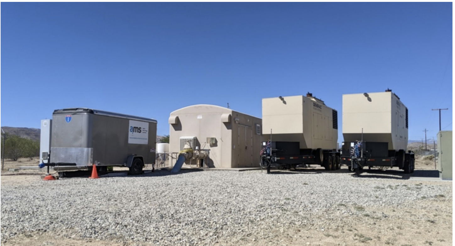
Figure 1. SafeGuard™ H2O Cr6 Removal Demonstration Trailer at Joshua Basin Water District. The demonstration system was comprised of five main components: the stannous reagent generation control module, electrolytic reagent generator, contactor, sand media filter and the MetalGuard™ online Cr6 monitor.
