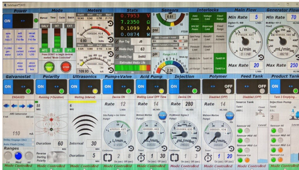
Figure 2-7 SG-H2O Pilot System HMI
