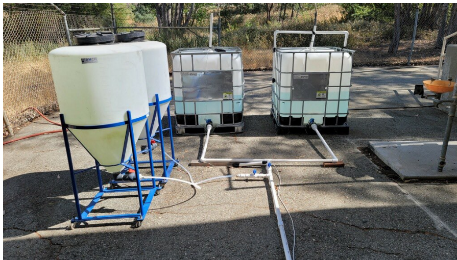
Figure 3-4 Initial Feed Water Tank System Configuration
