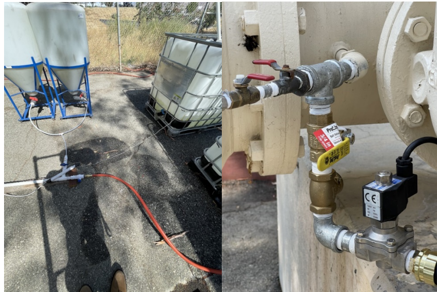
Figure 3-5 Totes Disconnected and Direct Plumbing Installed
