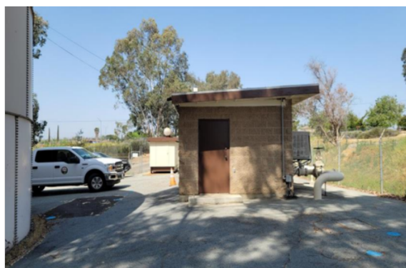
Figure 3-2 Well C2 Building
