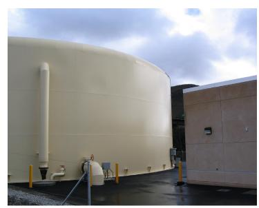
2 MGD storage facility (Clearwell #2) at San Luis Obispo Water Treatment Plant where the online THM-100 is used to control the TTHM removal equipment.
