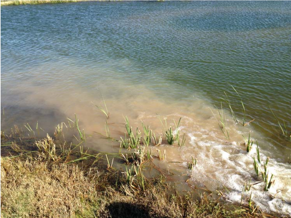
Figure 3-2 Discharge of clearwell solids into WTP backwash water lagoon
