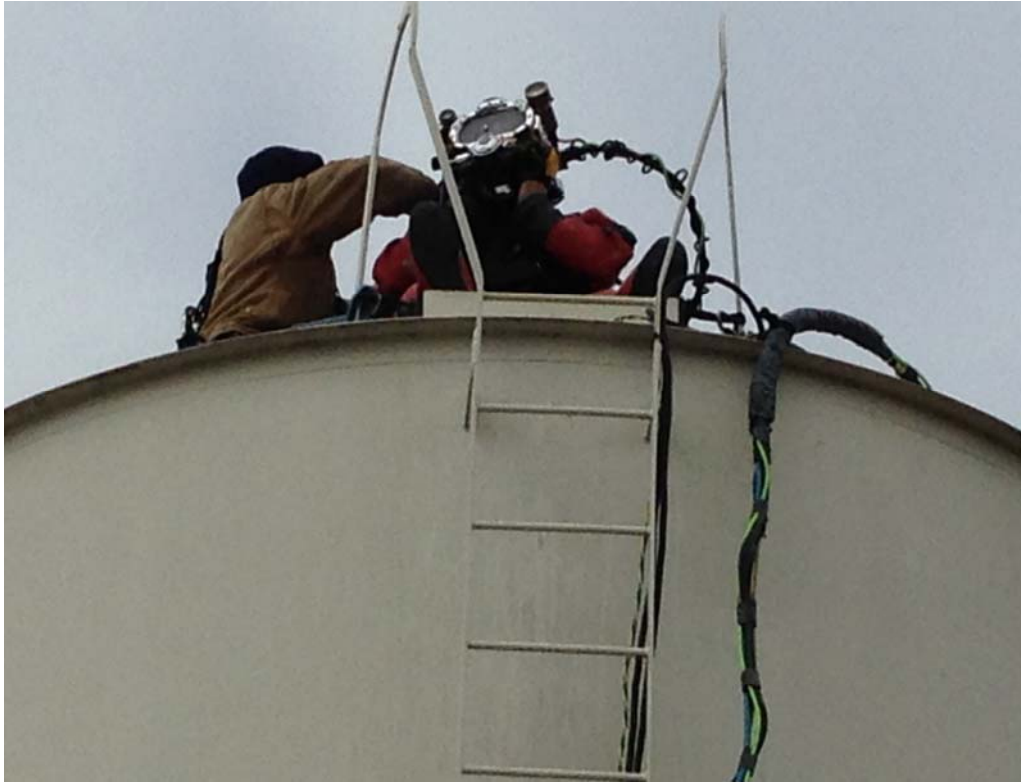
Figure 3-3 Diver in suit and helmet prior to entry inside the clearwell
