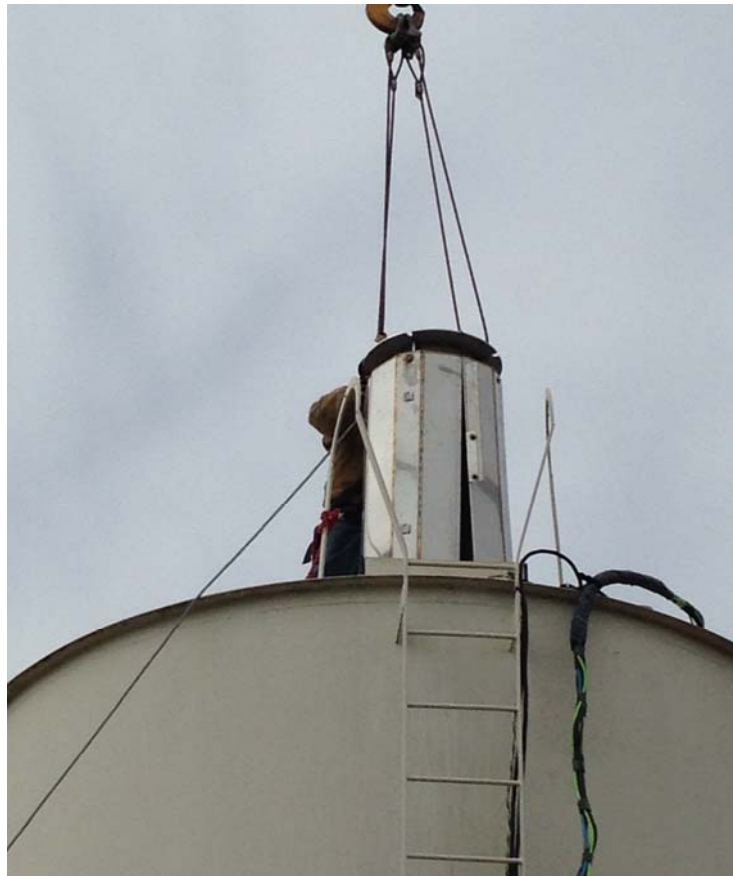
Figure 3-5 Surface aerator float being lowered into the clearwell using boom truck
