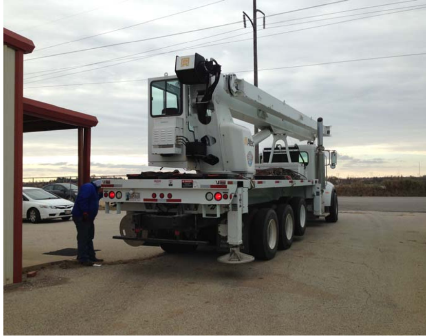
Figure 3-4 Boom truck set up during aeration equipment installation
