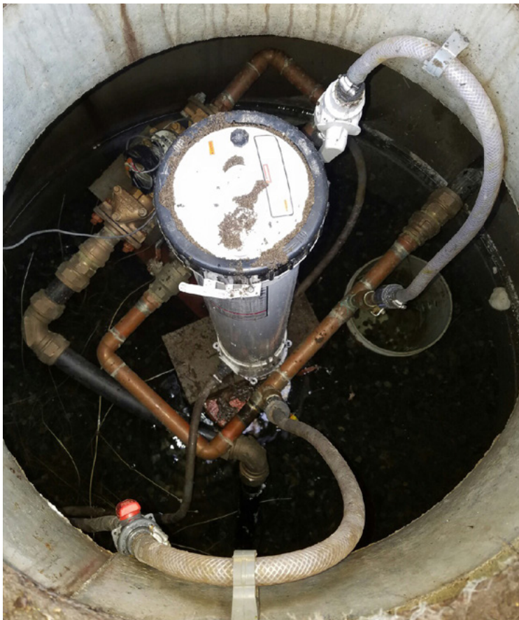
Figure 3: Typical Bleeder Vault Installation
